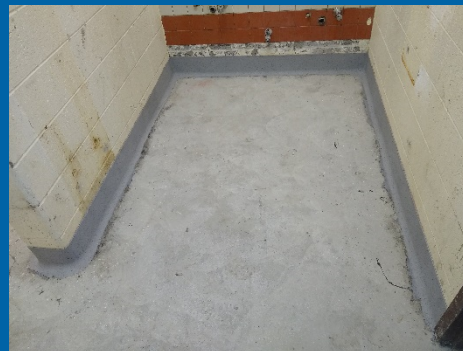
Begin installation of epoxy floor in restrooms at building 2020 and 2021
