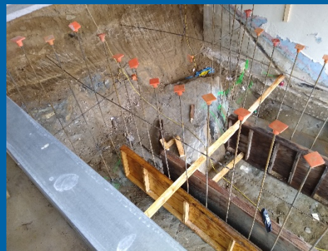
Drill and epoxy rebar at entrance
